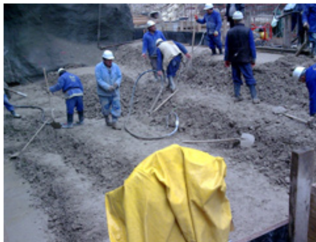
Figure 6: Placement of mass concrete
