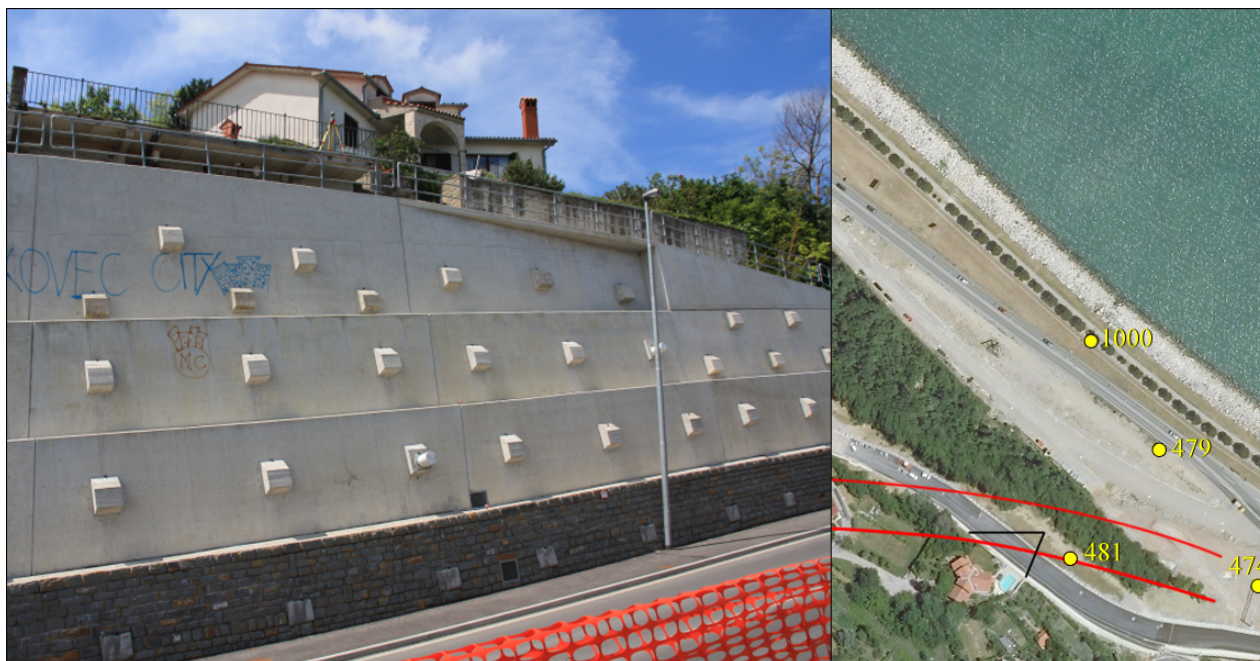
Figure 41: Objects of interest and stabilized pillars in Sector 1. Only about 25 % of the entire wall can be seen which stretches about 130 m in length and 10 m in height. The black line in the right image indicates the field of view of the left image.
