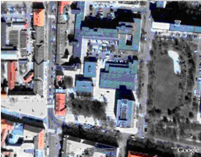
Figure 14 and 15: Master plan and satellite photo of the 'new' town centre institutional-ensemble [Korbonits, 2010, Google.earth].
