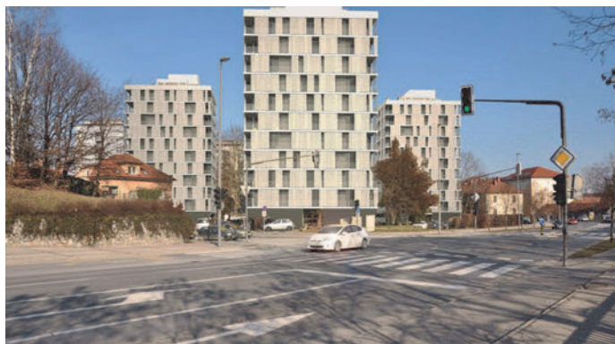
Slika 7: Pogled na stolpnico po sanacijskem posegu. Figure 7: Tower building after proposed reconstruction.
