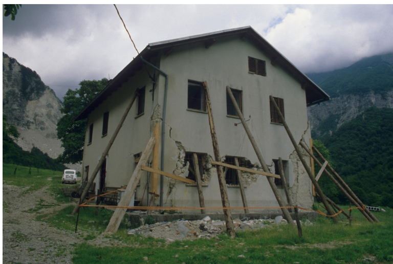
Fig. 1. In 1998 earthquake mainly older buildings, built of rubble and simple stone, were damaged (left), but also several monuments (right) (photo: A. Gosar).
