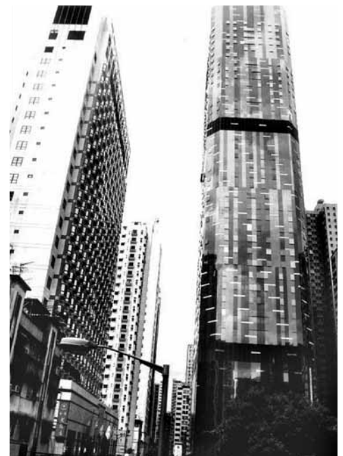
Stolpnica AIA, Hong Kong, 1999. AIA Tower, Hong Kong, 1999.
