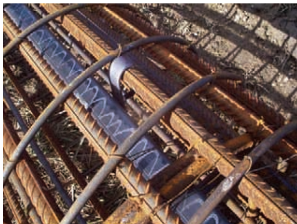
Figure 8. The measurement channel fixed between the reinforcement of the pile.
