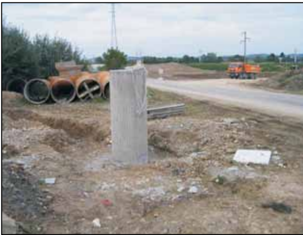
Figure 6. The top of the testing pile before the installation of the loading equipment.
