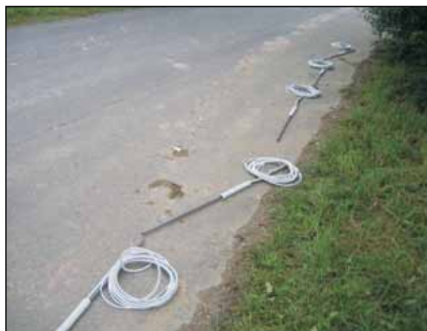
Figure 3. Finished sensors prepared for installation in the pile reinforcement.
