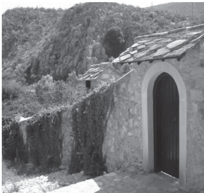
Slika 5: Vhodna cesta v stanovanjski kompleks. Figure 5: Entry road to a residential complex.
