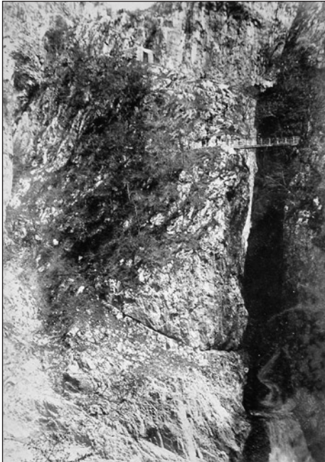
Fig. 24: The Tommasini bridge at the side of Navavni most (phot. Benque on f.4).
