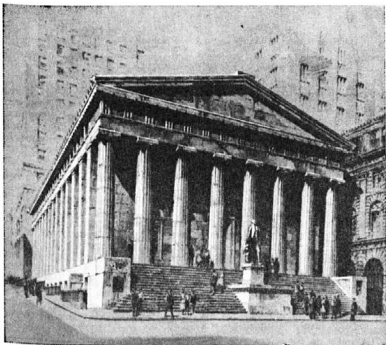
Federal Hall v New Yorku.
