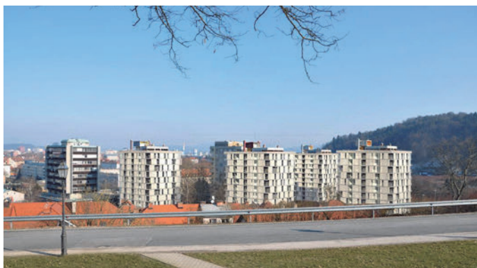
Slika 8: Panoramski pogled na stolpnice po sanacijskem posegu. Figure 8: Scenery view of the tower building after proposed reconstruction.
