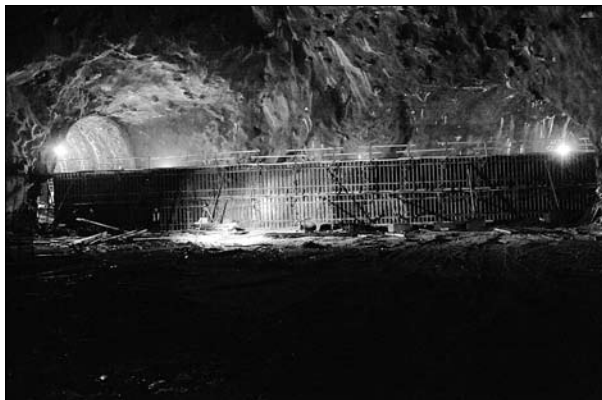
Fig. 11a: Constructing bridge in cavern (Photo: M. Garašić).
