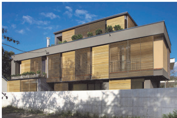
Figure 4: First finished building (one-family house) with 'seismic foundation pillow' in the world.
