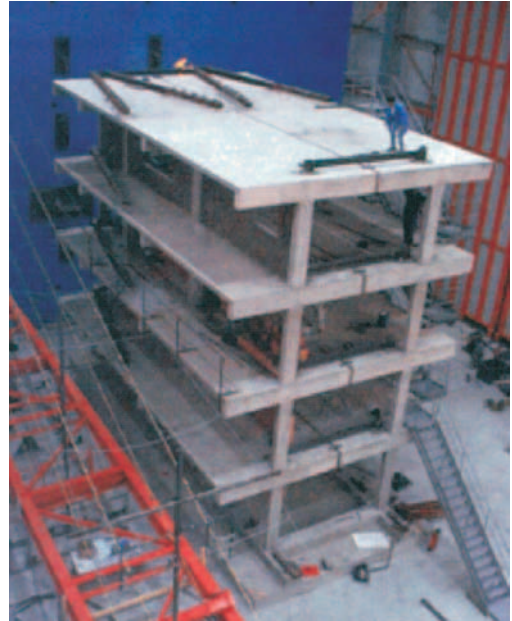
Figure 2. The four-storey reinforced concrete frame building which was tested at ELSA Laboratory
