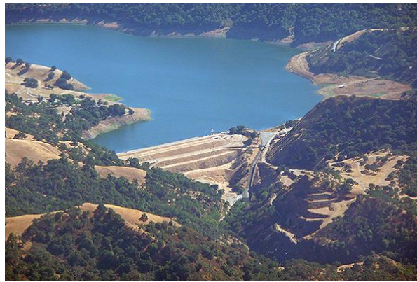
Stara pregrado bodo nadomestili s kombinirano nasuto (vir: https://www.water-technology.net/projects/calaveras-dam-replacement-project/ )
