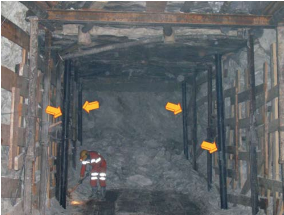
Figure 1. View of a drift supported by timber sets and hydraulic (arrows) and mechanical props
