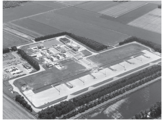
Fig. 12. Aerial photo of one gas production cluster near a canal. The wells surface at the light-grey rectangular area. The gas is treated in a plant before it is supplied to the international gas distribution network.
