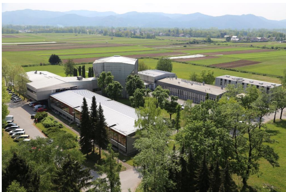
Figure 23: View of the IJS Reactor Infrastructure Centre
