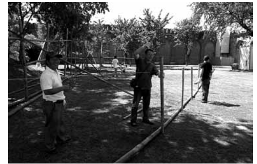
Gradnja v Benetkah. The construction process in Venice.
