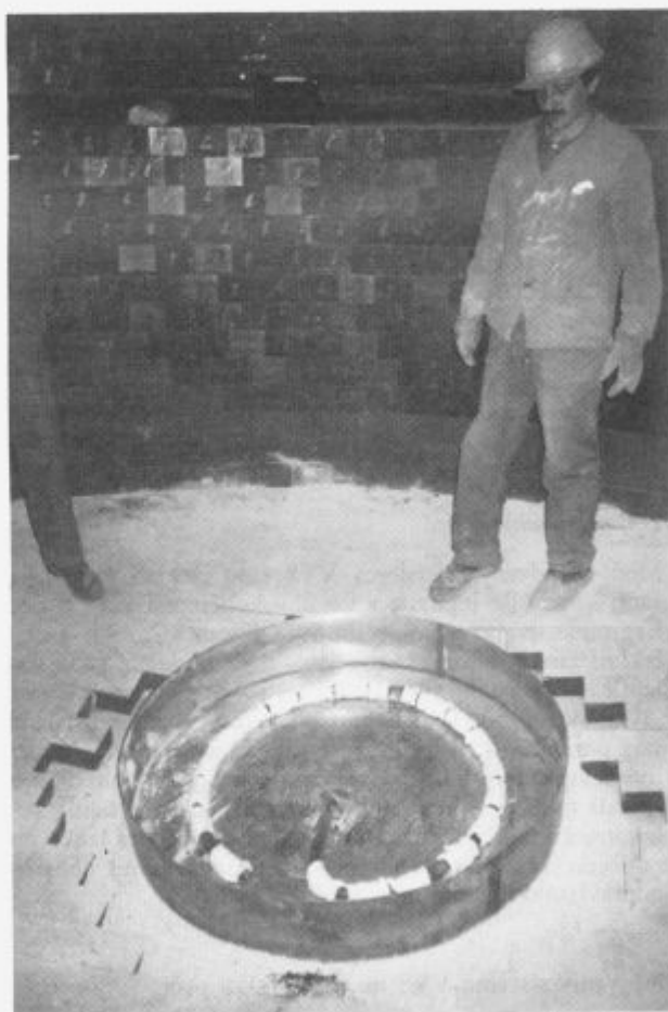
Slika 1. VVS element pred phanjem dna peči. Figure 1. Position of the VVS stirring element before bottom ramming.
