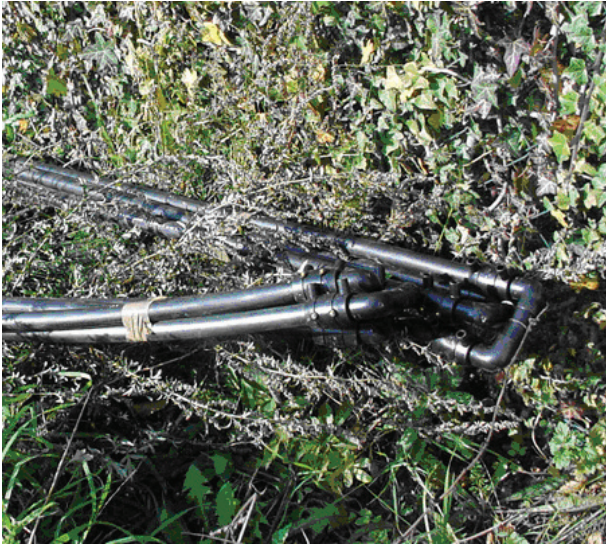
Figure 11. Detail of Fig. 10 showing the U-shaped toe zone of absorber pipes.
