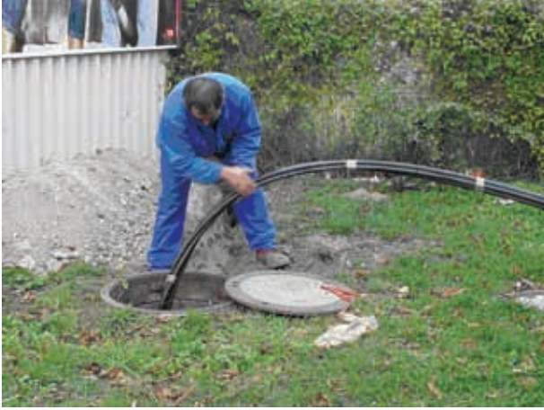
Figure 10. Installation of absorber pipes into the filter pipe of a well used for groundwater lowering during a cut and cover tunnel construction.
