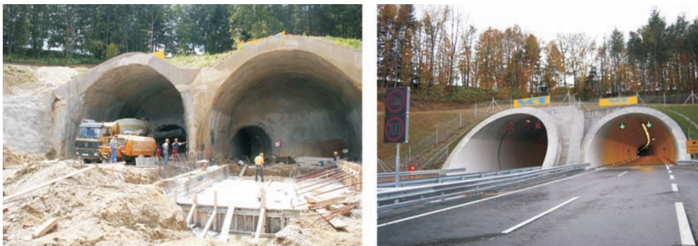
Figure 14. Tunnel Cenkova in phase of construction and after it on operation
