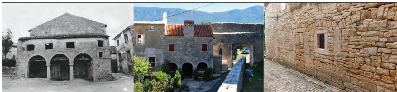
Fig. 9: Loggia in Tinjan, Kršan and Boljun, photo: I. Huic.
