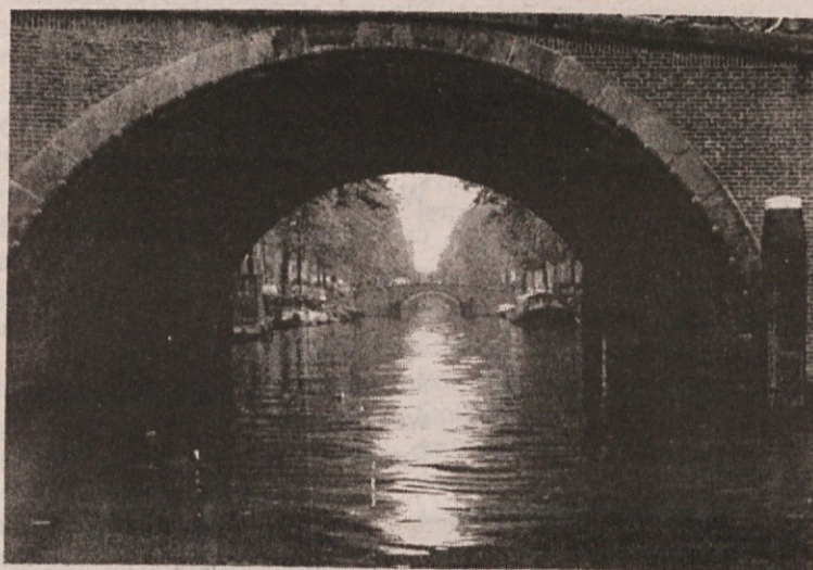
Bridges frame a canal in Amsterdam.
