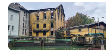
↑ As a result of the fire, the Sava hydroelectric power plant will not operate for the time being, while its rehabilitation will be expensive and long-term Photo: Elektro Gorenjska archive
