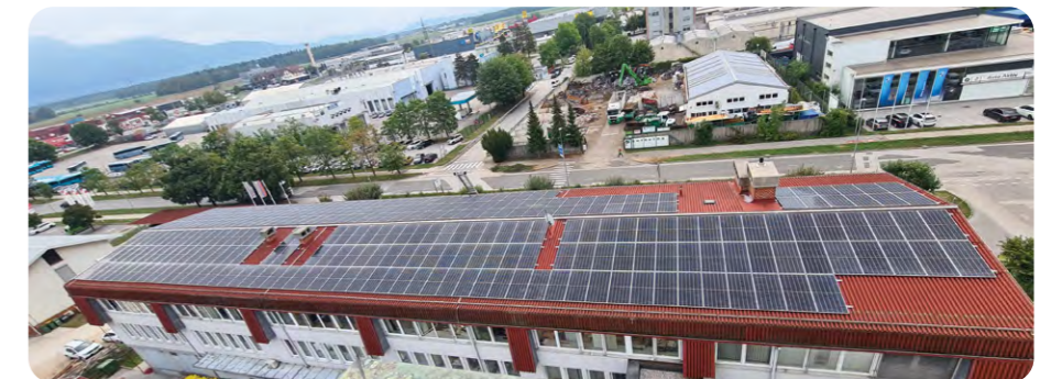
↓ Solar power plant on the old building of the company Elektro Gorenjska Photo: Robert Jošt
