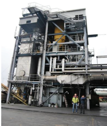
Figure 2: Gasification tower Güssing, Austria
