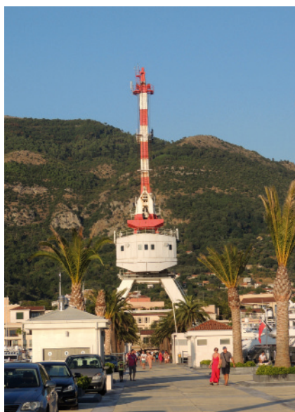
Figure 4: Crane Jetty 1, reminiscent of Sava Kovačević – Arsenal as the symbol of Porto Montenegro.
