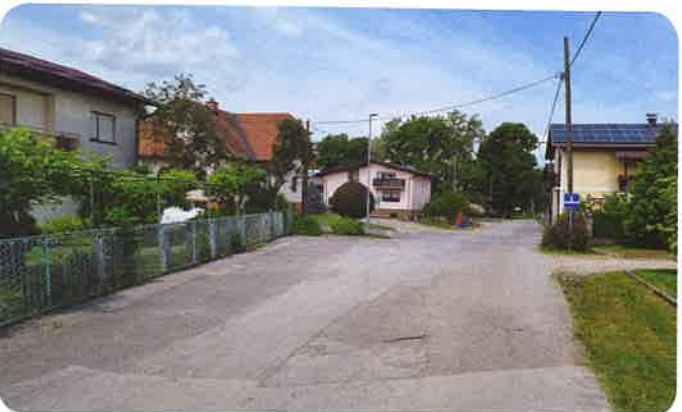
Rekonstrukcija ceste in vodovoda v Zg. Jablanah 26, 24, 25, 23, 21, 22, 20 in 19a
