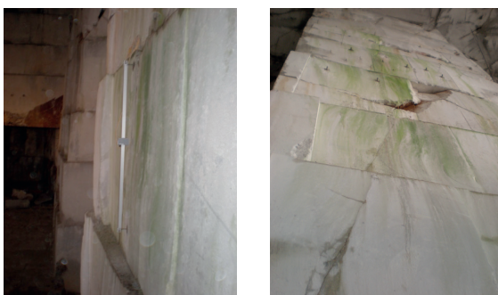
Figure 5: EL beam gauge on the high safety pillar VS3.
