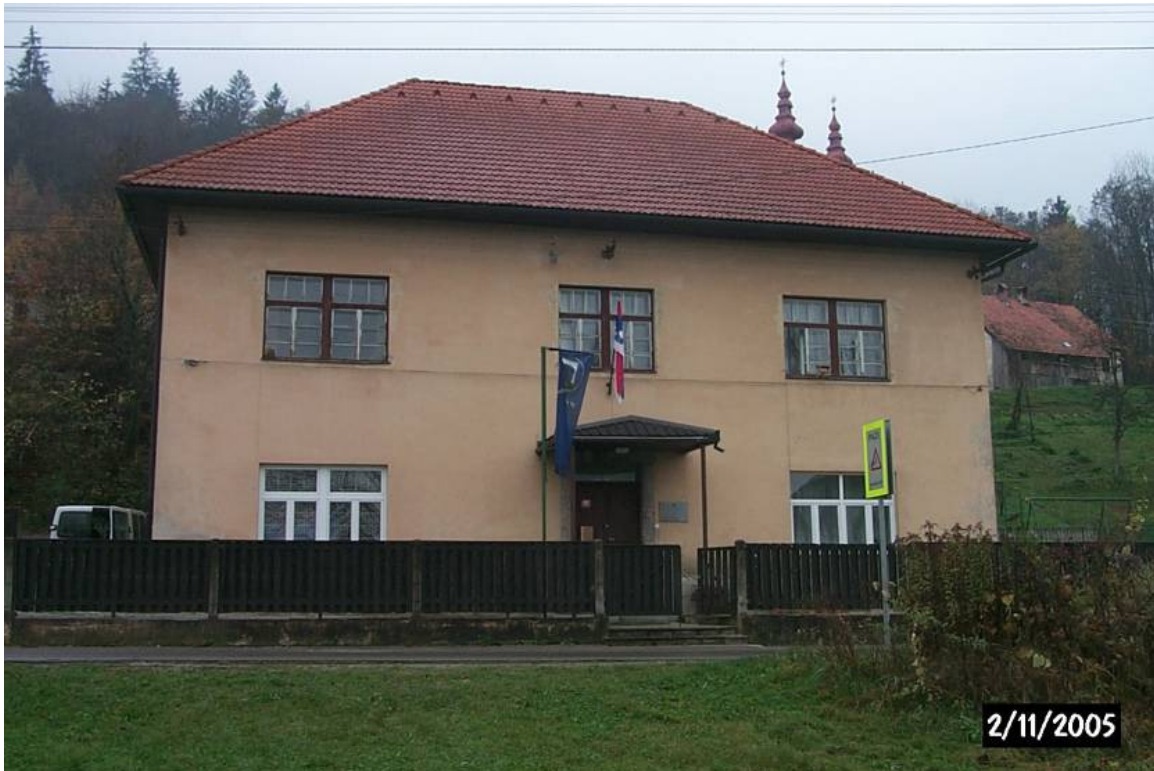
Slika 22: Osnovna šola Tomišelj – severna fasada Figure 22: Primary School Tomišelj – northern facade
