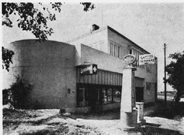
Ing. arch. N. Dobrović, Prag Vila lekara, pogled
