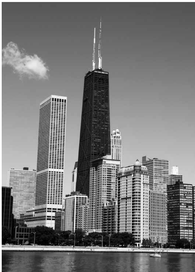
Slika 12: John Hancock Center arhitekturnega biroja Skidmore Owings & Merrill LLP, in Water Tower Place biroja Loeb, Schlossman & Hackl. [Vir: http://www.flickr.com/photos/brostad/4750924251/sizes/o/in/photostream/ ].
