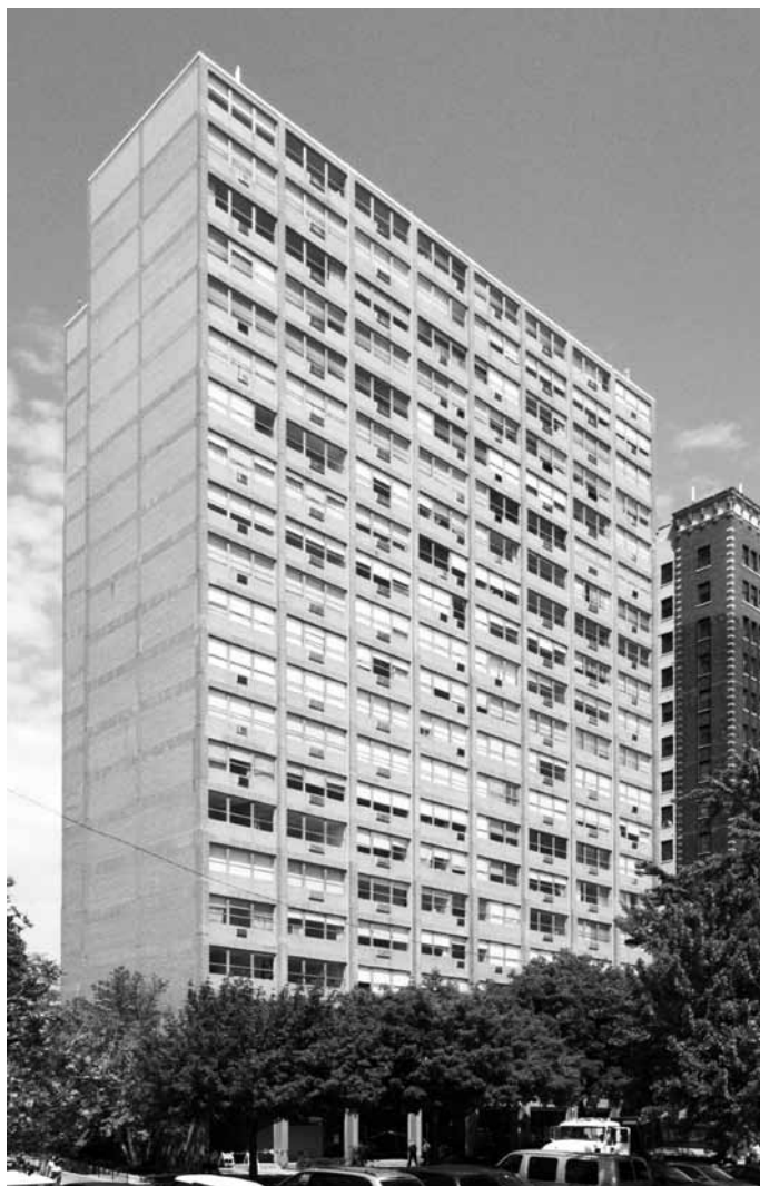
Slika 1: Mies van der Rohe: Promontory Apartments, 1949. [Vir: http://archiveofaffinities.tumblr.com/post/5972225050/mies-van-der-rohe-commonwealth-promenade ].
