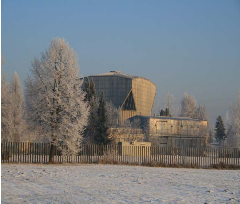
Figure 23: View of the IJS Reactor Infrastructure Centre
