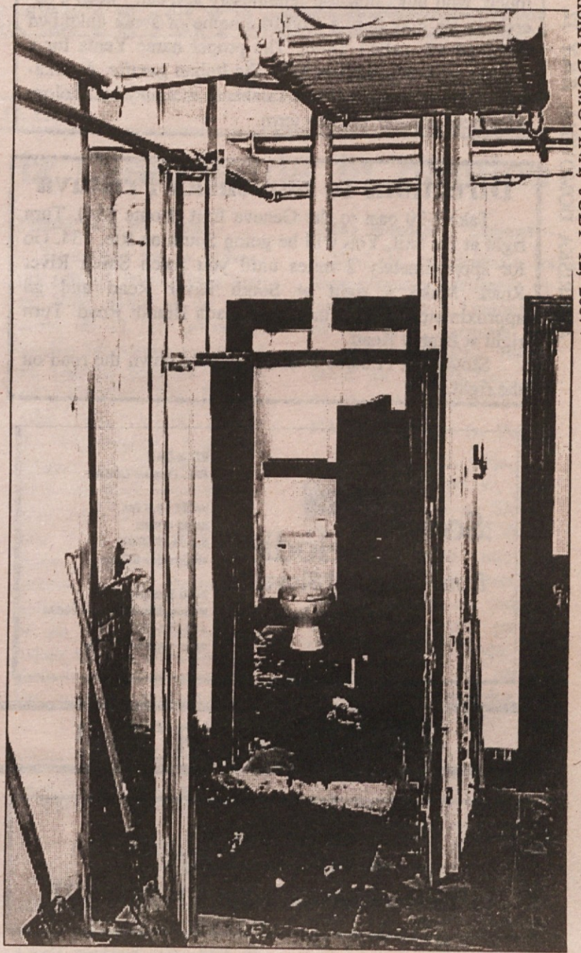
Restroom in St. Vitus church basement gets much-needed renovation.
