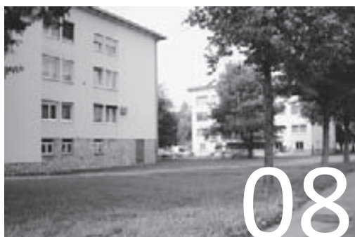
Stanovanjski bloki_ 1956–62_ Ulica Štefana Kovača 1-21
