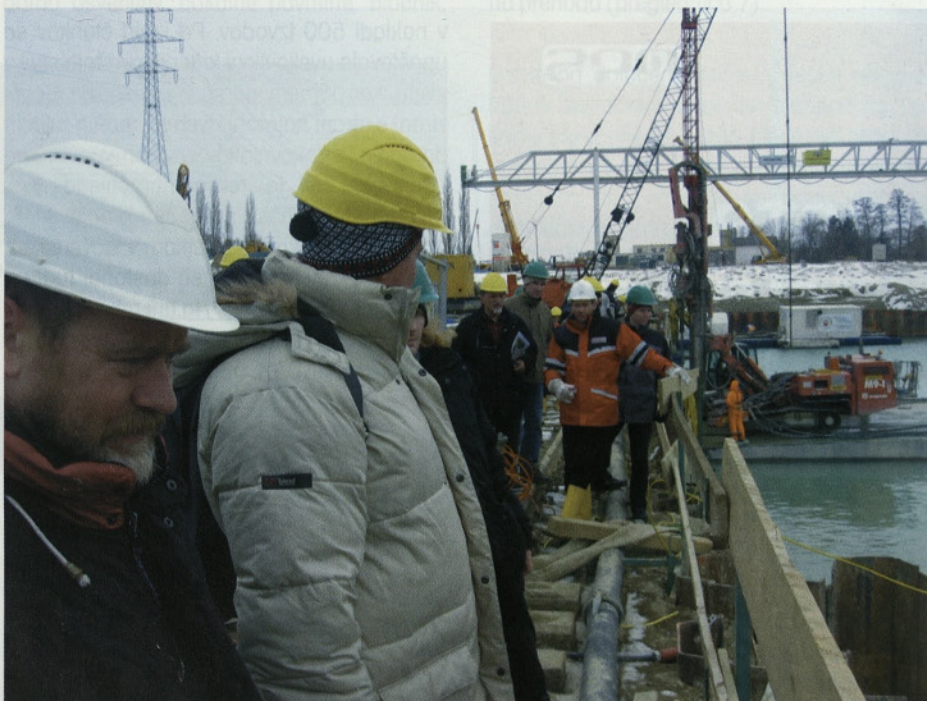
Ogled gradnje tunela S1 Tunnel Rannersdorf, Schwechat
