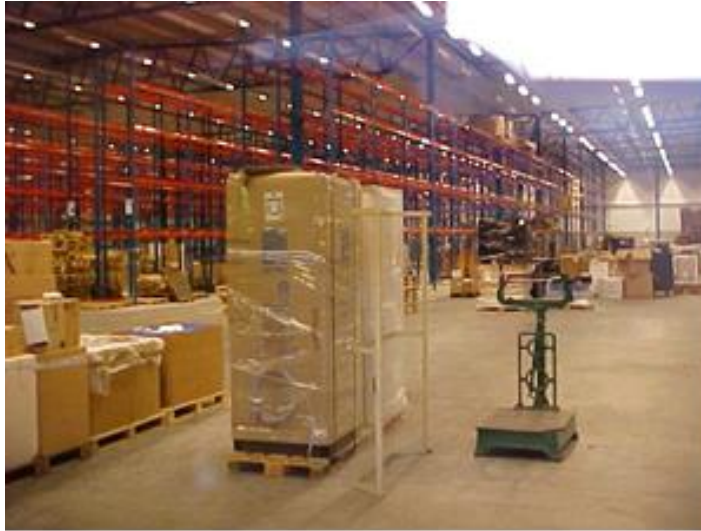
Figure 12. Example of an industrial concrete floor in a storage building. Photographer: J. Hedebratt.
