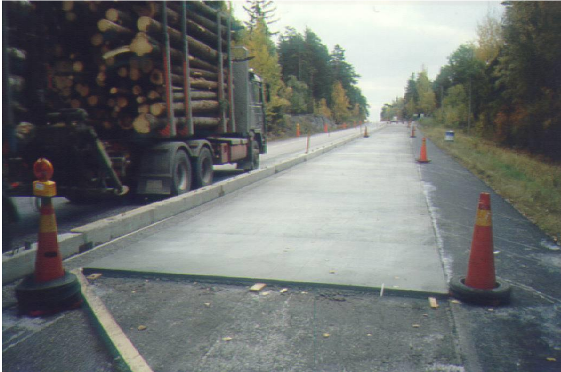
Figure 14. Whitetopping. Steel fibre concrete overlay on an old asphalt road (Silfwerbrand, 1995).
