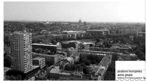
Poslovna zgradba Adris, Zagreb, natečajni projekt. Adris group Building, Zagreb, competition project.
