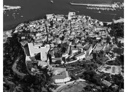
Osnovna šola Frana Krsta Frankopana, Krk, 2003, pogled iz zraka Aerial view of the Elementary School Fran Krsto Frankopan, Krk, 2003.
