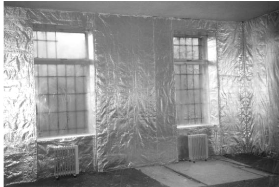
Fig. 3. Reference room on the 2 nd floor of the SEM building heated with conventional radiator system
