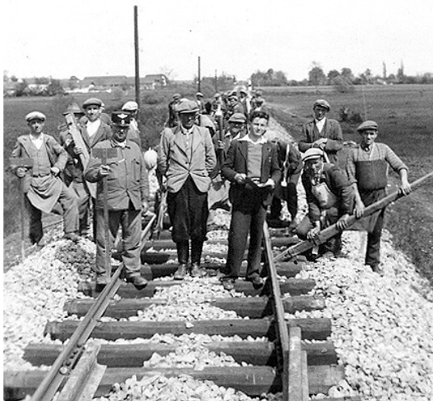
Fig. 9: Laying railway tracks near Hodoš in 1941.
