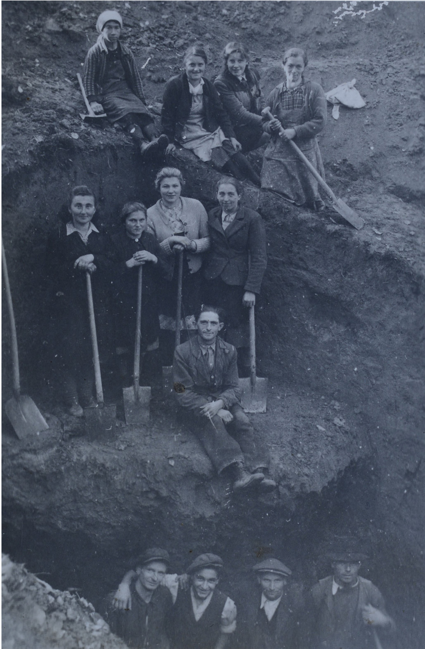
Fig. 5: The German defence line was built mostly by forcibly mobilized locals. The photograph shows a bunker that is being dug at Vonarje near Rogaška Slatina.
