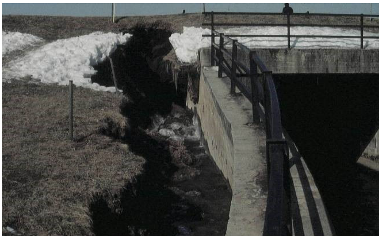
Figure 8: Dam collapse due to internal erosion along the spillway.
