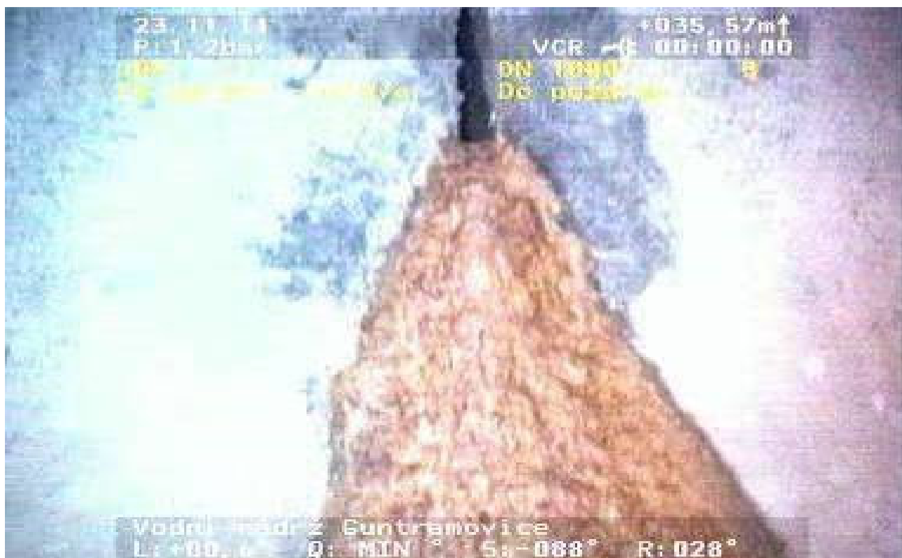
Figure 7: Crack in the bottom outlet pipe with turbid seepage into the pipe.
