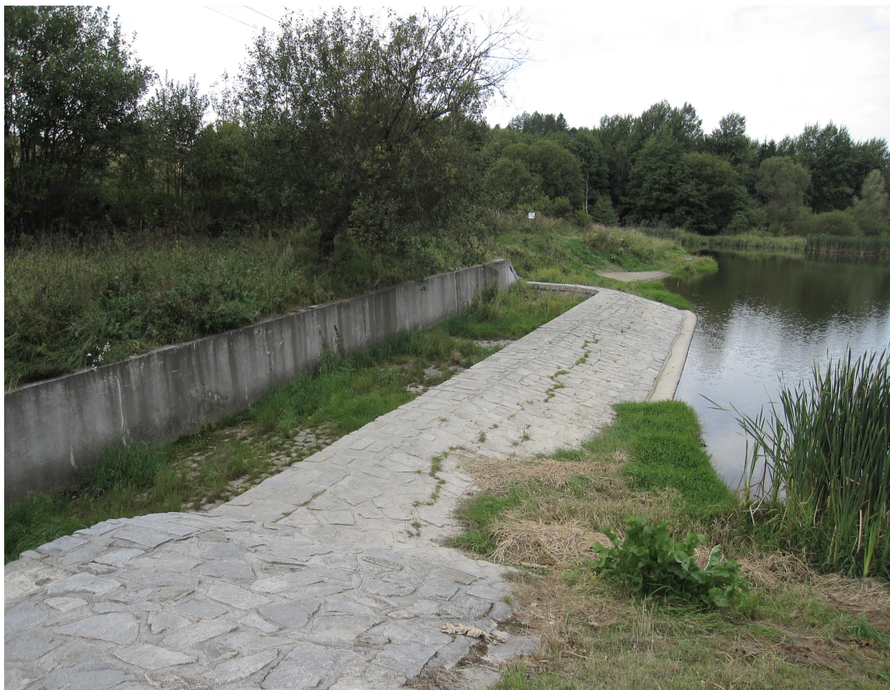
Figure 9: Long, shallow and narrow spillway channel affected by sediment and vegetation.
