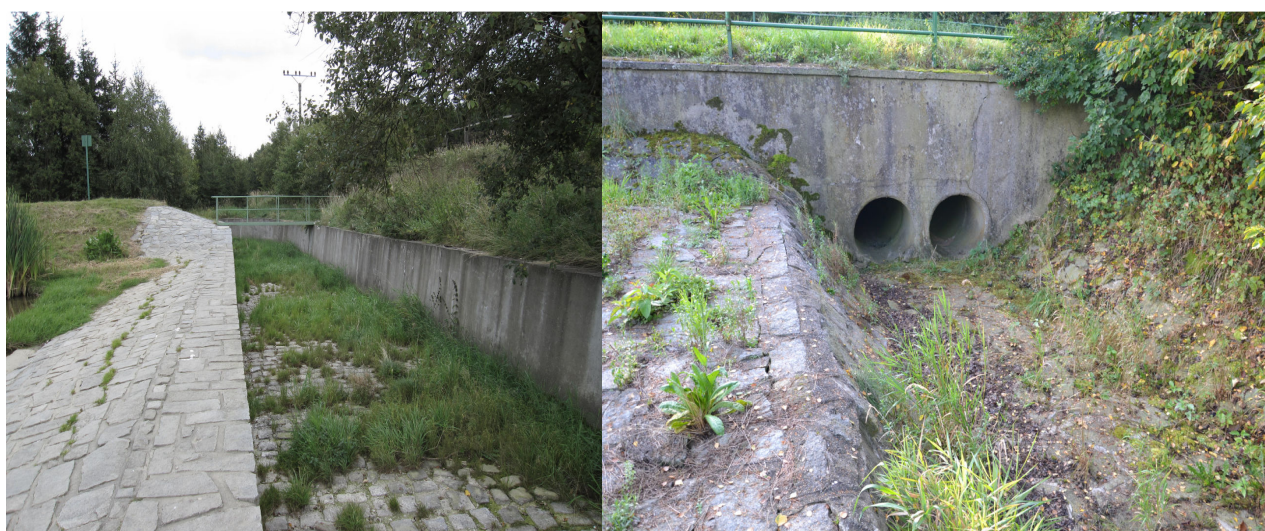
Figure 10: Crossing of the spillway chute with the dam by a narrow bridge (left) and culvert (right).
