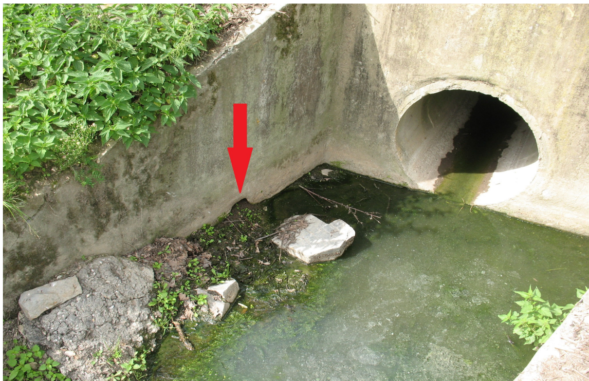
Figure 6: Low downstream end of a bottom outlet with submerged drain pipes (arrow).
