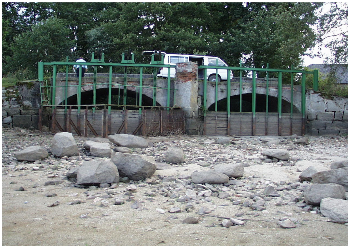
Figure 5: Gated sluice with damaged propulsion equipment.
