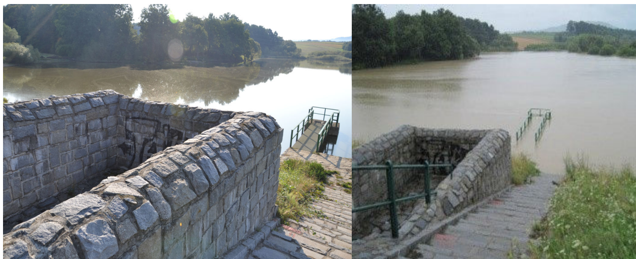
Figure 3: Submerged bottom outlet entrance and its operation during a flood.
