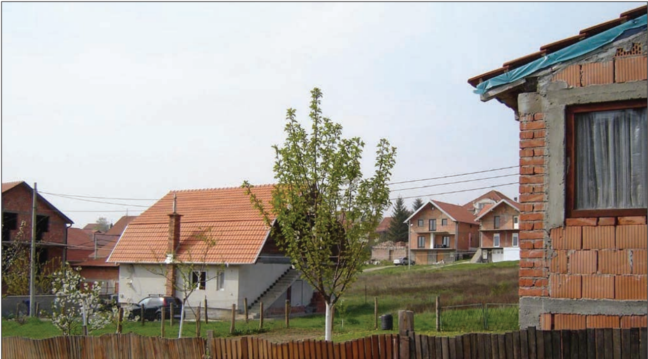
Figure 2: Kaluderica – suburban (peripheral) area of Belgrade
