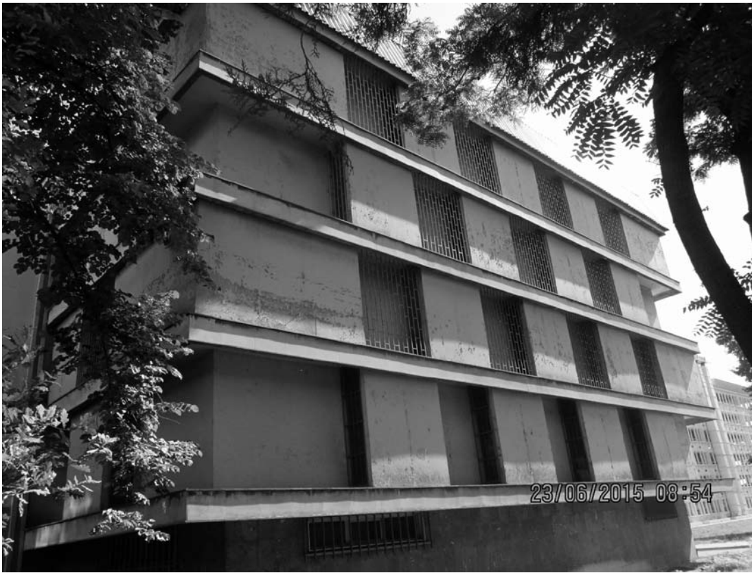
Picture 2. The old repository of the State Archives of the Republic of Macedonia
