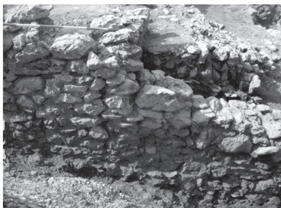
Sl. 2.50: Severna cerkev, stik zidov 1 in 21 – zunanje lice. Fig. 2.50: North church, the contact of walls 1 and 21.
