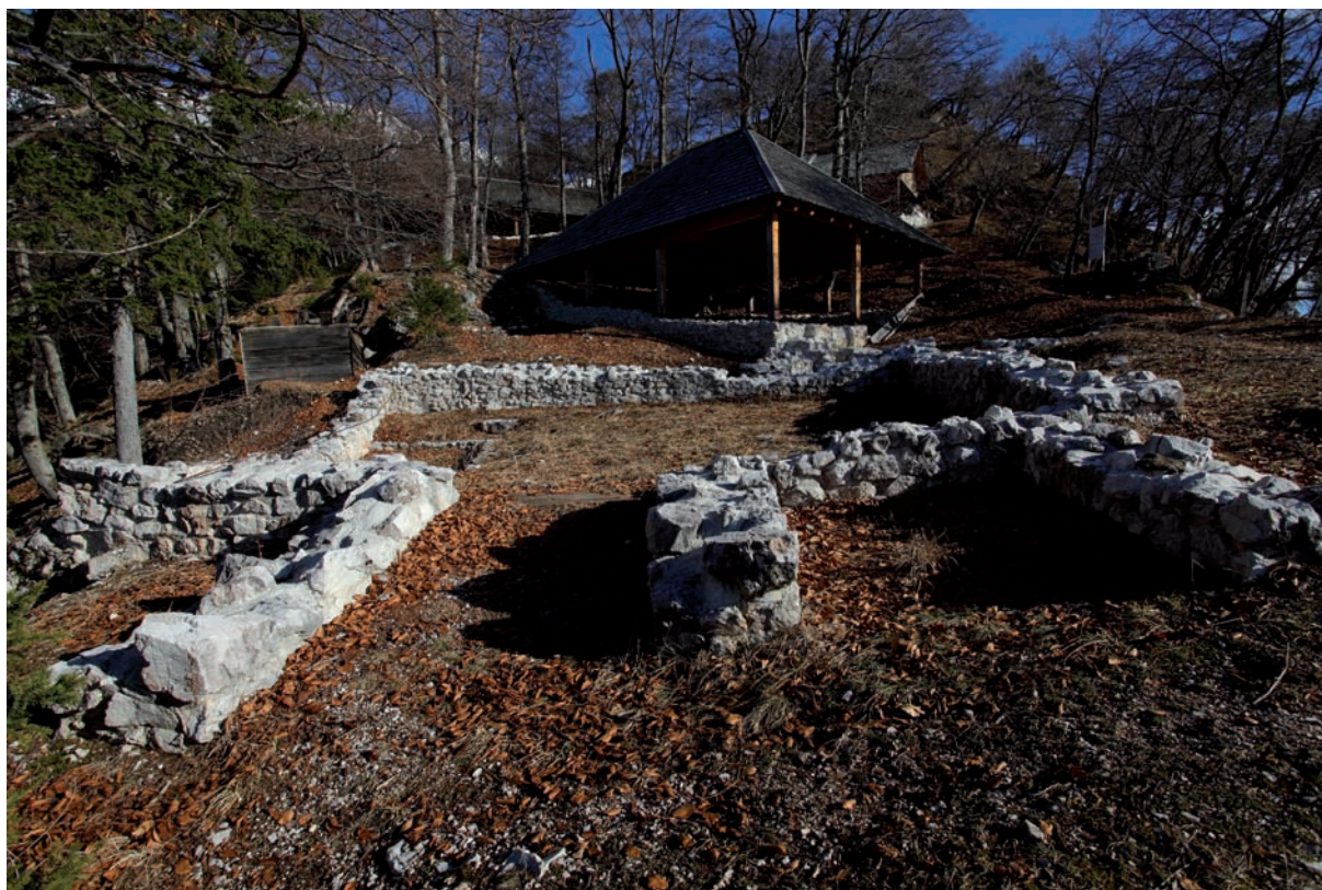
Sl. 4.3: Ajdna nad Potoki. Konservirani ostanki zidane zgradbe z dobro vidnim vetrolovom na južni strani naselbine. Fig. 4.3: Ajdna above Potoki. Preserved remains of the building with a wind shield on the south side of the settlement.
