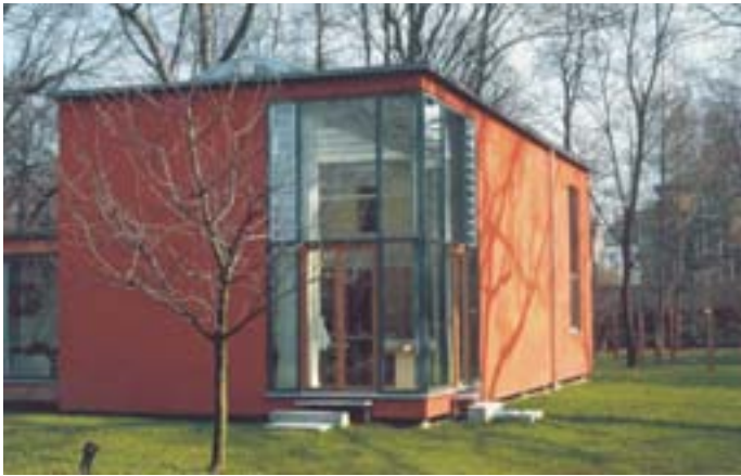
Slika 11: Kiparski atelje – zasteklitev na južni fasadi, stena je obdelana z apnenim ometom [Vir: Zogler, 2004:22]. Sculptor's atelier – glazing on the south facade, the wall is finished with lime plaster
