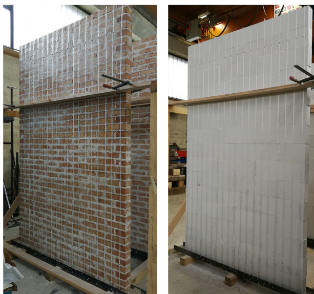
Slika 5.11: Utrjen NF preizkušavec (levo) in YT preizkušavec (desno) s sistemom C. Figure 5.11: Strengthened NF specimen (left) and YT specimen (right) with strengthening system C.
