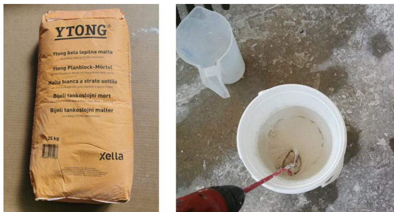
Slika 4.16: Pakiranje tankoslojne lepilne malte (levo) in njena priprava (desno). Figure 4.16: Bag of thin layer adhesive mortar (left) and its preparation (right).
