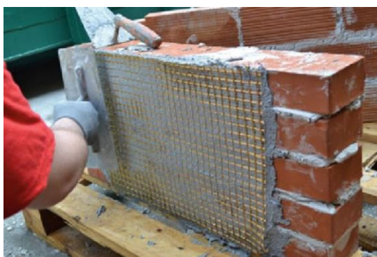
Slika 2.11: FRCM utrditveni sistem (Calabrese et al., 2020). Figure 2.11: FRCM strengthening system (Calabrese et al., 2020).
