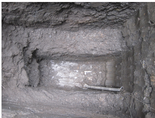
Fig. 3. Trial pit for performing falling-head test (photo: Zmago Bole).
