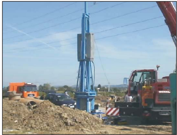
Figure 7. The testing site during the dynamic load test.
