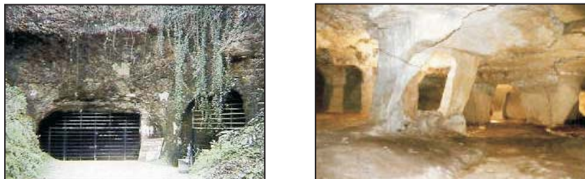
Figure 1., 2. Underground excavation of natural stone at the old Beer quarry [11].
