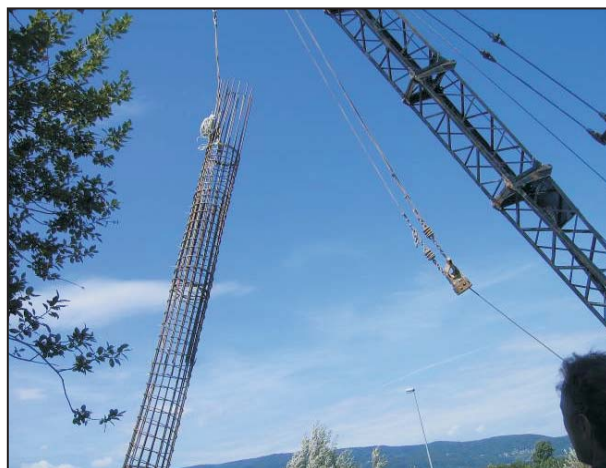
Figure 5. Placing the pile reinforcement equipped with nine strain sensors into the pile pit.
