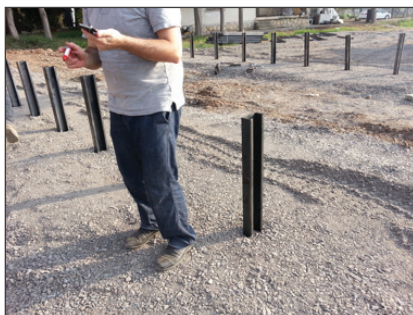
Figure 4. Installation of posts in soil.
