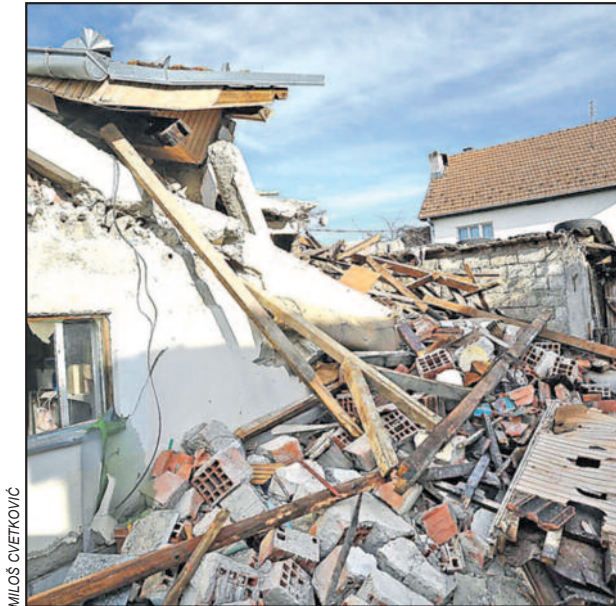
Aftermath of the Kraljevo earthquake.
